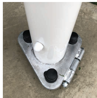
Hinged steel baseplate onto which the non rotating flagpole is fixed.
