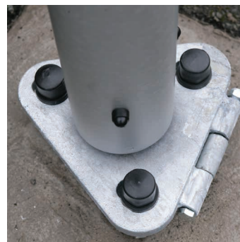
Hinged steel baseplate onto which the substantial rotating bearing unit is housed.
